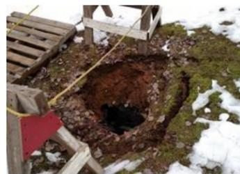
Hole in the Ground from Collapsed Septic Tank
